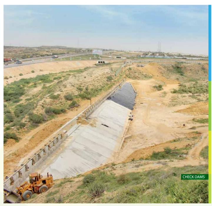
Dams have been constructed in DCK where accumulated rain water is stored which goes down in the soil and in this way the Aquifer is refilled and recharged by the accumulated water thus the underground water level is maintained. Five Check Dams have been constructed in DCK for accumulation/storage of rain water and for constant recharging of Aquifer to maintain the underground water level. In this way constant Aquifer recharging phenomenon is ensured.
