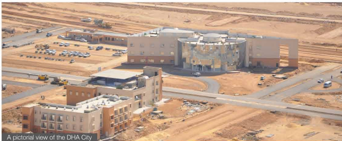
Another view of fast pace development work
